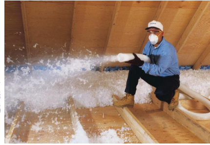
Above, from left rim joist insulation, rafter vent properly positioned and insulated, illustration showing proper attic venting system, and loose fill blown-in insulation in attic rafters.
